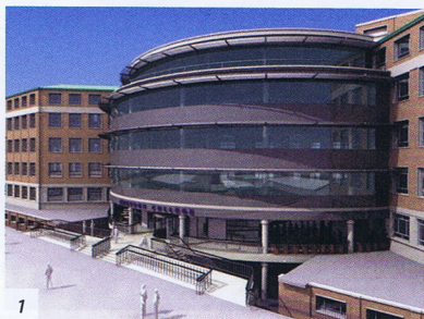
The completed rotunda (1) will house a new entrance hall (2) and the structure features CHS columns (3) which will remain exposed
